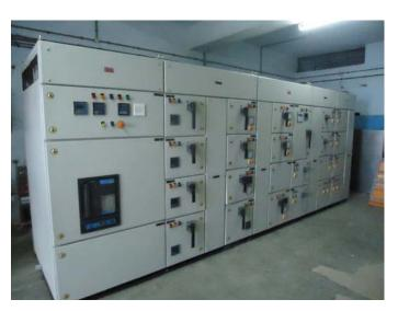
intelligent MCC which can communicate with PLC, can be start and stop from SCADA, you can measure its power parameters from control room.
